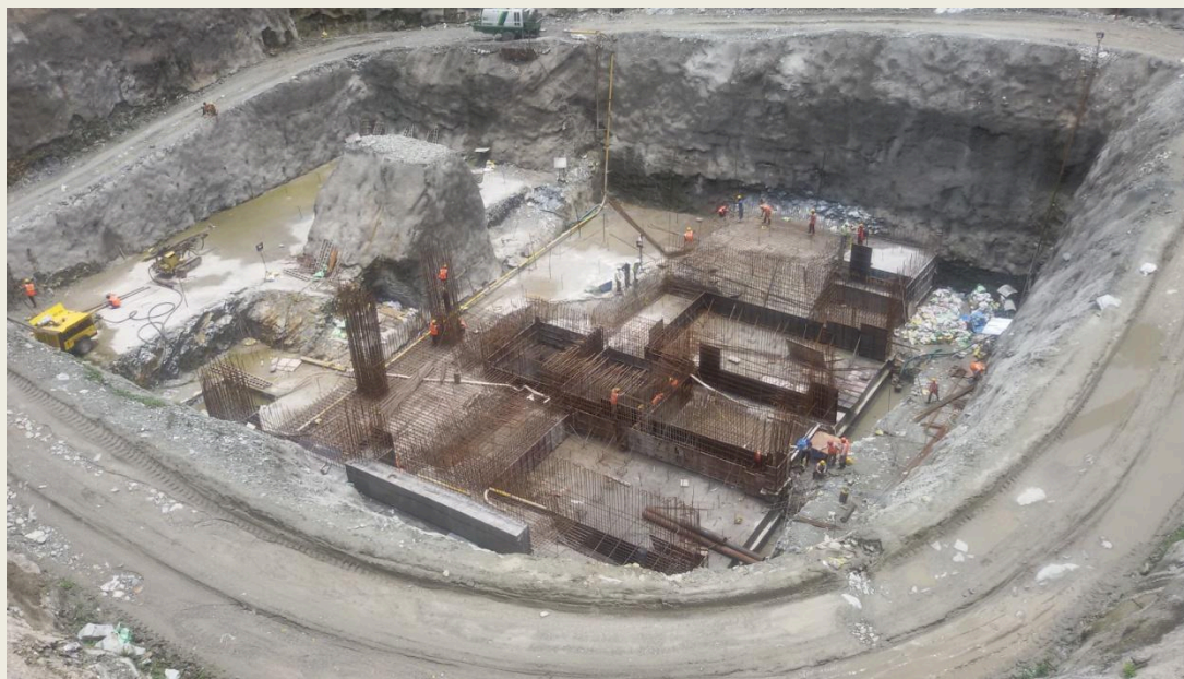
View of under-construction Powerhouse of 96 MW Tashiding HEP.
