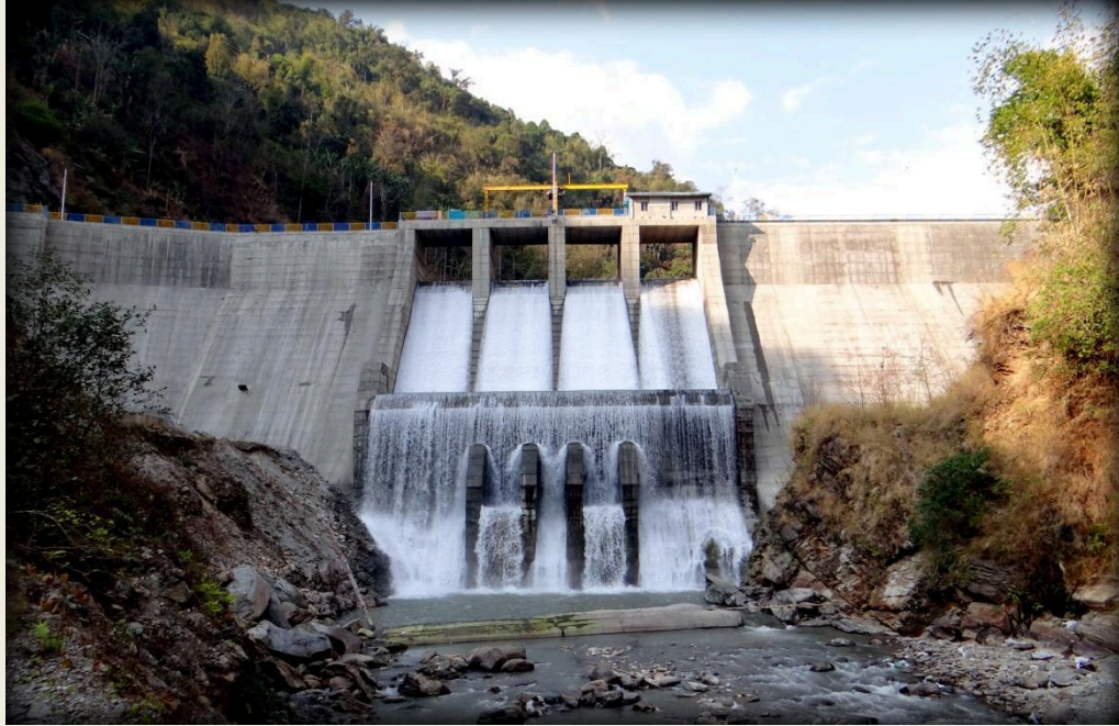
Rangpo Dam of 99 MW Chuzachen HEP(Source- M/s Gati Infrastructures Ltd).
