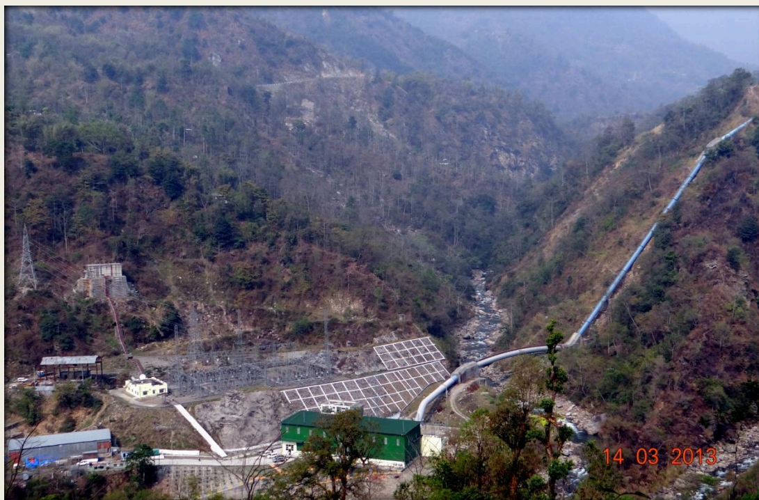
View of Power House and Penstock of 99 MW Chuzachen HEP
