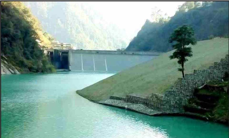
Dam and Reservoir of 1200 MW Teesta-III HEP
