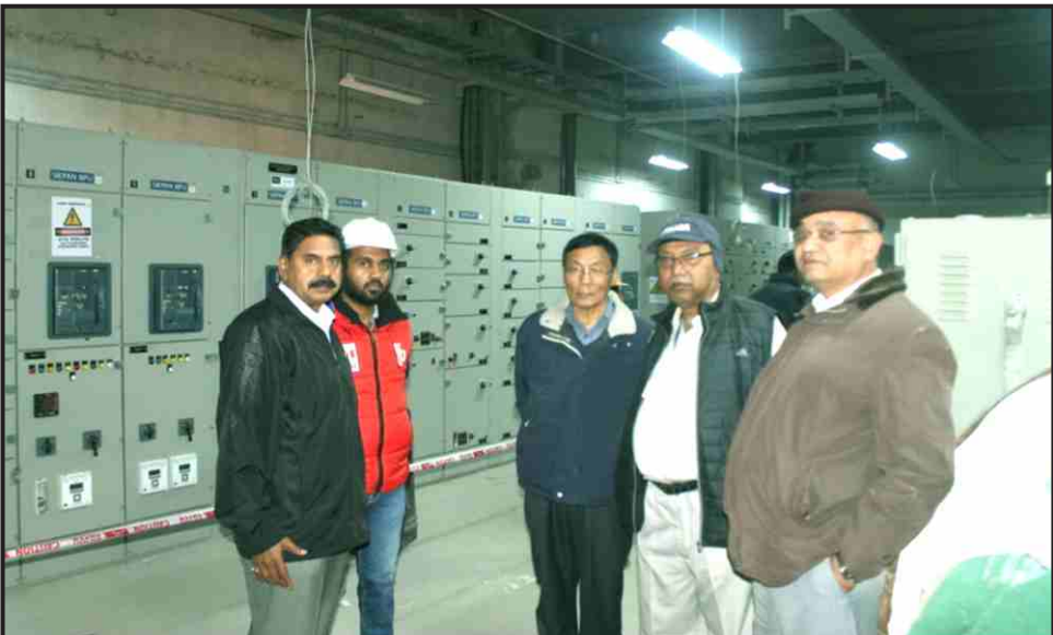
At the Powerhouse of 97 MW Tashiding HEP.
